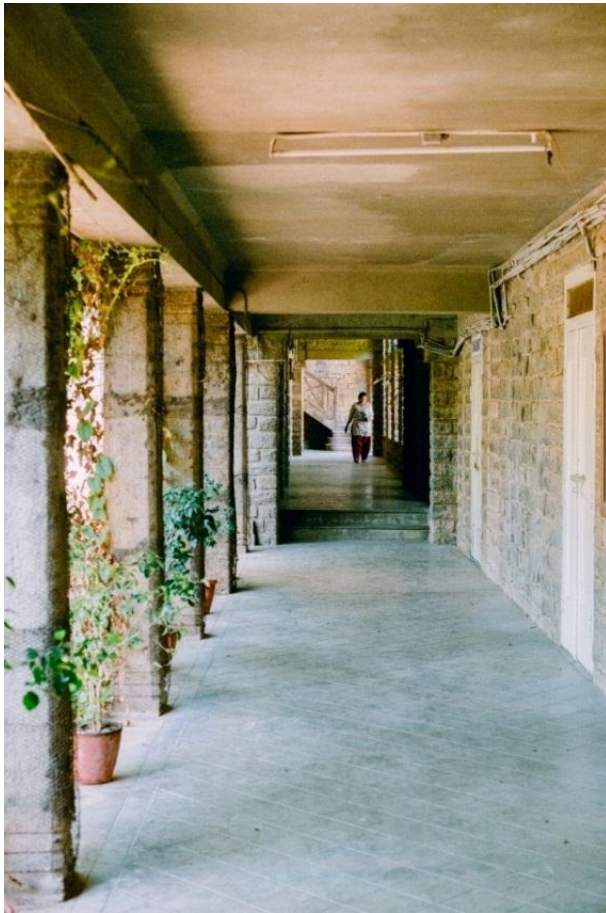
Stone corridor in front of the chapel
